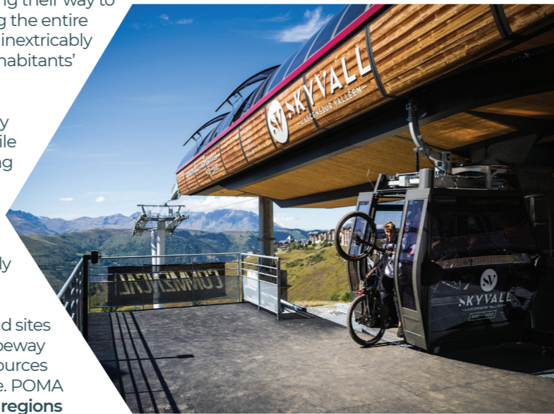
SKYVALL Valley Lift - Loudenvielle - FRANCE - 2019
